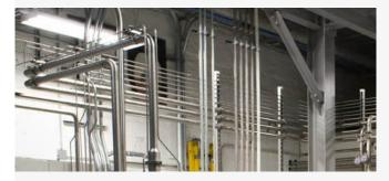
Design/Build extension of a stainless steel purified water distribution loop to connect to two new production lines and related CIP and COP systems.
