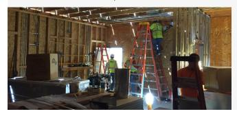
Kroeschell constructed an 800-sf. kennel and storage facility, installed a new AHU, and connected new equipment to existing BAS while also installing new DDC controls. Additional square footage improved the environment of care, ensured compliance with regulations, and met all health and safety standards.
